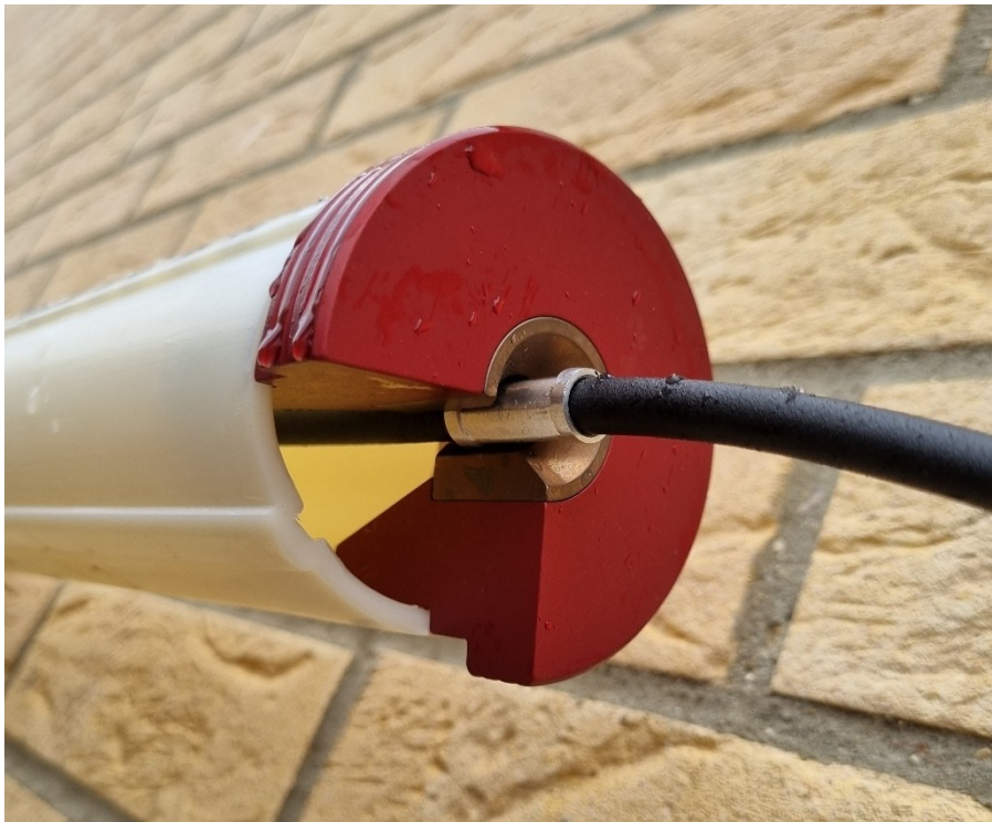
Figure 23: Cable gate fitted onto the access end of the casing
