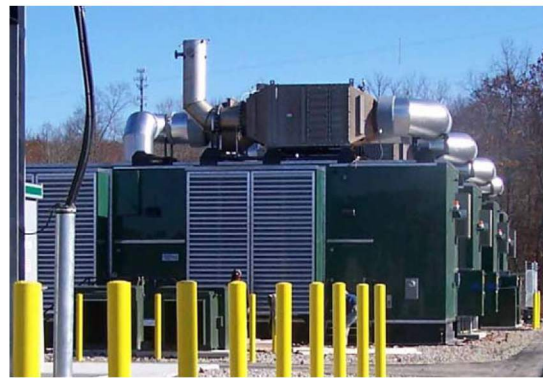
SCR Installation
